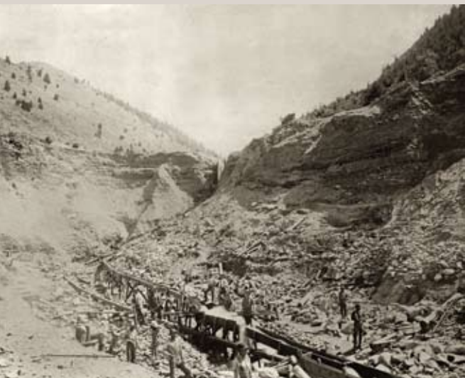
FIGURE 6.23: When all the easy gold was taken, miners turned to larger-scale operations. They built wooden flumes to transport water from a nearby creek. The water poured through a sluice box, where it washed the heavy gold from dirt and gravel. Think of all the shoveling it took to placer mine this way.
