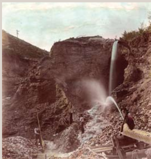
FIGURE 6.24: Hydraulic mining tore apart the landscape. Water from a high-pressure hose blasted dirt, gravel, and gold into a sluice box. The hose was connected to a flume, which brought the water to the claim from a nearby creek.
