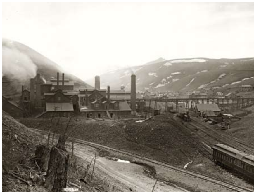
FIGURE 9.14: Railroad transportation helped silver smelters like this one at Wickes grow into large, industrial complexes. These towns offered thousands of jobs to newcomers.
